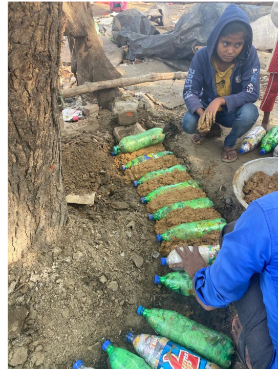
In Ayodhya, India a Roots & Shoots school made eco bricks with plastic waste
